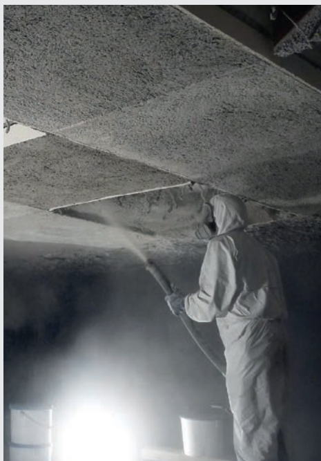
Shotcrete: 100% quality. Only 25% downtime.
