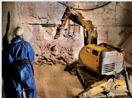
Safe & fast wrecking.
